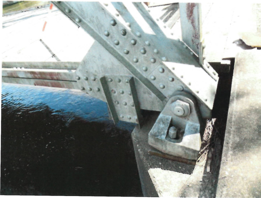
Photo 7 - Northwest Bearing at Abutment
