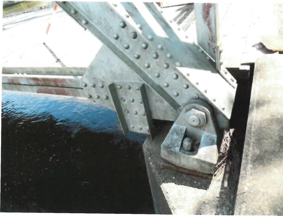
Photo 7 - Northwest Bearing at Abutment
