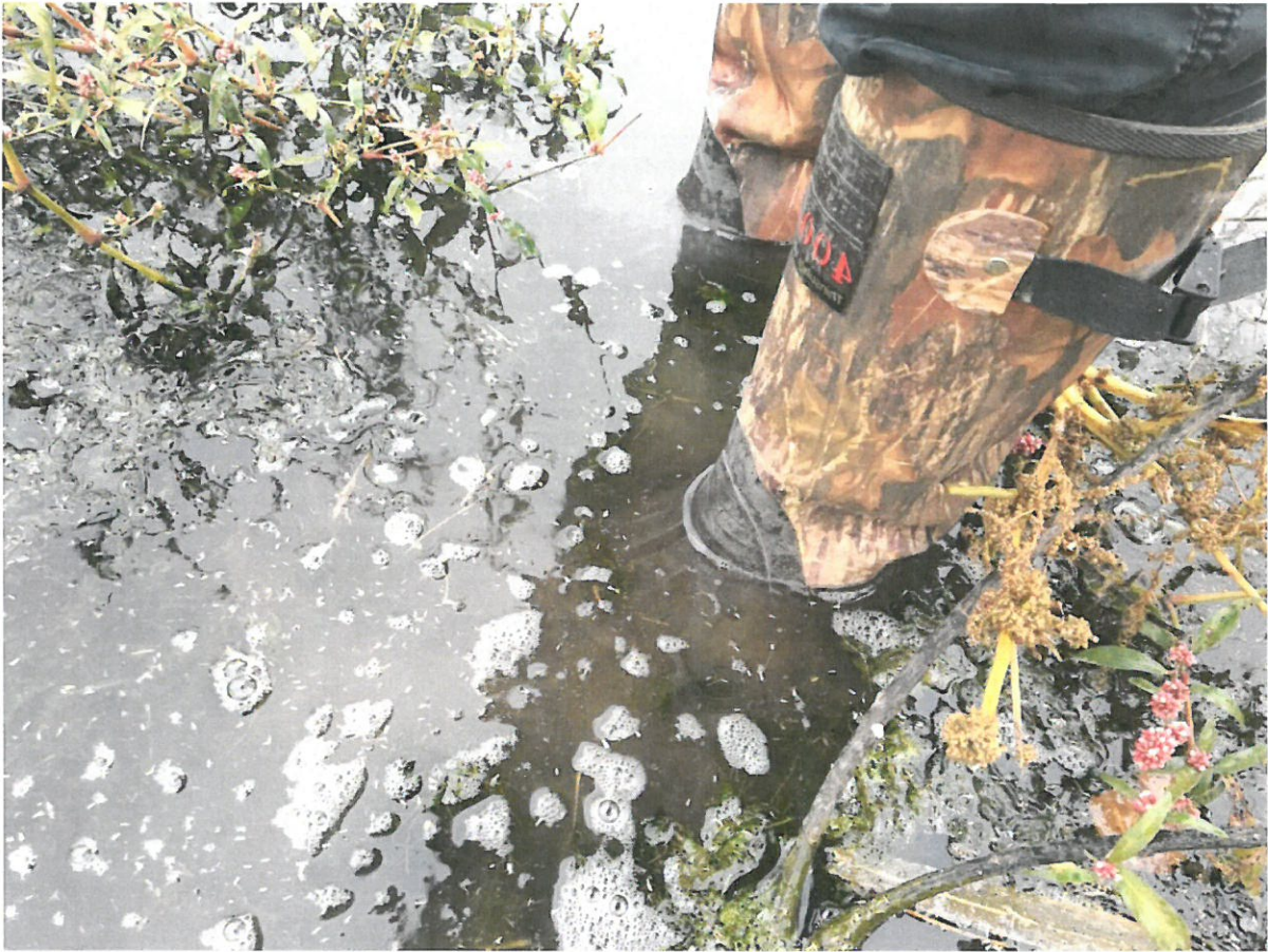
The standing water has to be 4"-6" deep in the area above the main. Clearly, not draining properly.
