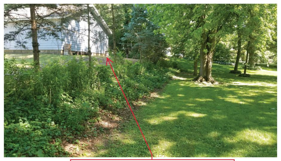
placement of fill to construct elevated pad for garage (height difference from bottom of slope to rear of garage is 5+ feet)
