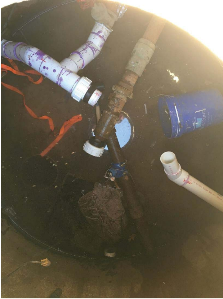
11/18/20 View of the pit next to the well where new distribution system piping and valves were in process of installation.
