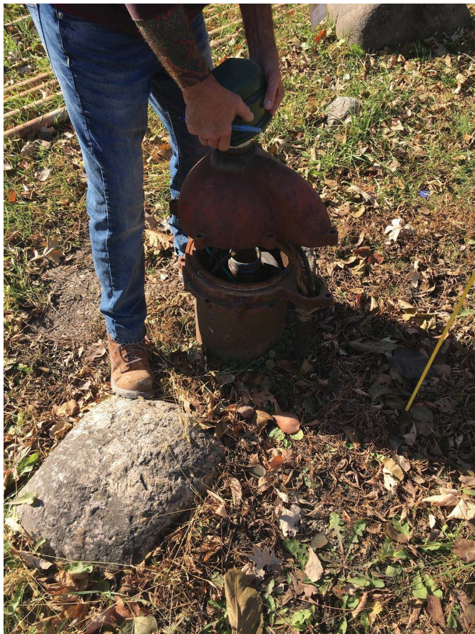
11/6/20 View of well cap without bolts, missing gasket
