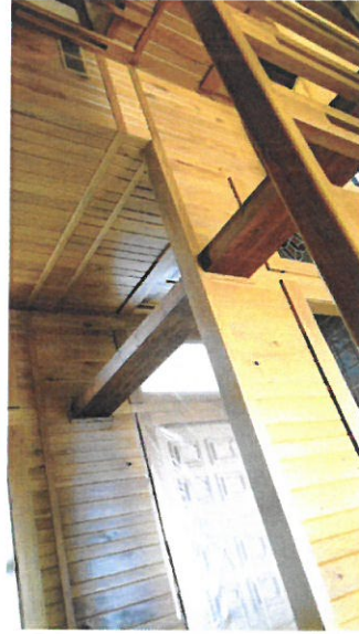
1. View located over existing open entrance way
