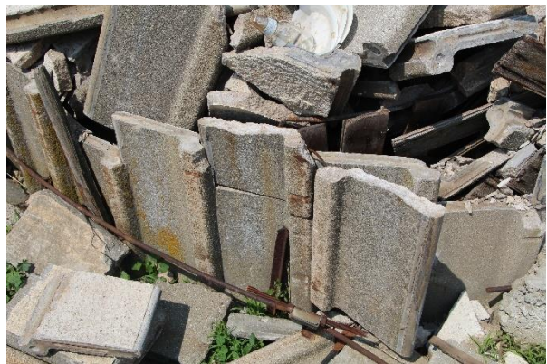
The two silos at the Coombs-Chally Farmstead, site 751, have collapsed, exposing the design of the concrete staves and steel hardware used in their construction.
