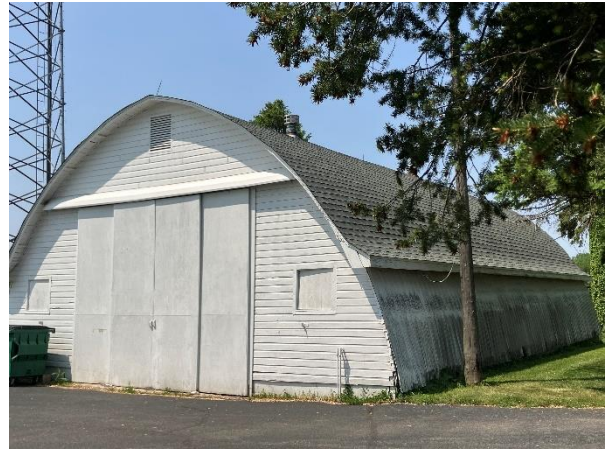
Left: The Quonset shed at Windett-Renton-Wallace Farmstead, site 523, is typical of this 1940s building type in the survey area. Right: A Quonset shed at Boomer-Holdiman Farmstead, site 2125, is a typical example of this building form built of wood-framed construction.
