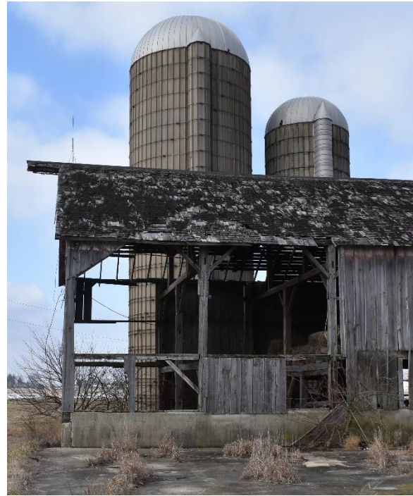
Left: A drawing of heavy timber barn framing from 1894 [William E. Bell, Carpentry Made Easy, or the Science and Art of Framing (Philadelphia: Ferguson Bros. & Co., 1894), plate 7]. Right: The loss of exterior cladding from this barn at the Knudson-Neusus-Phillips-Holt Farmstead, site 2851, has exposed its original heavy timber frame.
