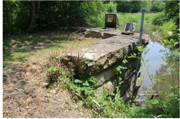
Left: The former farm road in Section 21 of Bristol Township, now called Boomer Lane, was bypassed when Illinois Route 47 was constructed. Right: On the north bank of Blackberry Creek, the limestone bridge abutments for this former road still exist.
