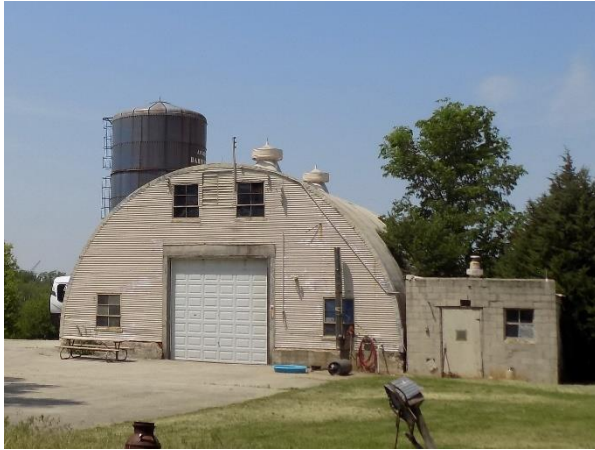
Left: The Quonset shed at Windett-Renton-Wallace Farmstead, site 523, is typical of this 1940s building type in the survey area. Right: A Quonset shed at Boomer-Holdiman Farmstead, site 2125, is a typical example of this building form built of wood-framed construction.
