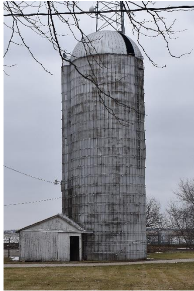
Examples of concrete stave silos in the survey area. From left to right, these examples are at the Wilkening-Thurow Farmstead, site 1752; Penman-Ament Farmstead, site 2152; and the Wheeler-Sullivan-Cazalet Farmstead, site 1923.
