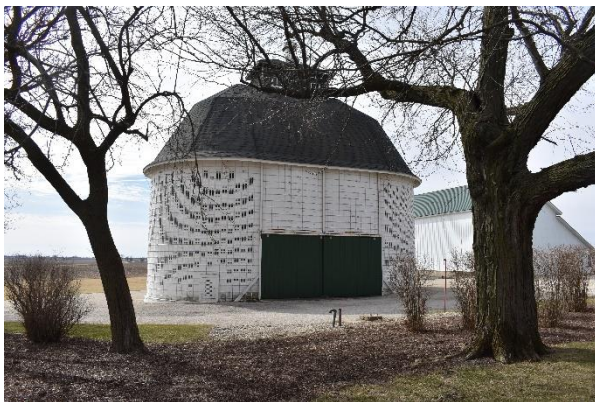
Left: The crib barn at the LeBaron-Roe-Campbell Farmstead, site 1154. Right: The crib barn at the Eglington-Egan-Undesser Farmstead, site 525. These distinctive rounded-end crib barns built using perforated concrete staves likely date to the 1940s or 1950s.
