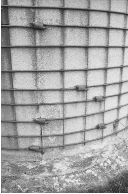
Above: A detail view of the steel hoops and turnbuckles on a concrete stave silo. Right: An advertisement for concrete stave silos from the Prairie Farmer's Reliable Directory (1918), 359.
