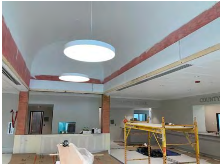
Flatstock trim being installed at lobby
