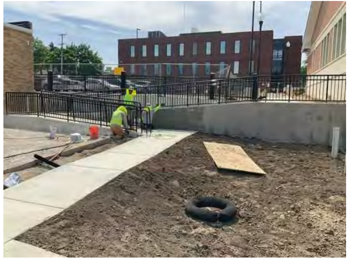
Rubbed finish install at ADA ramp
