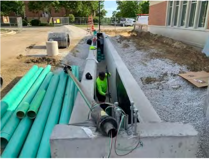
Planter box with waterproofing work Taken on May 31, 2024, 8:25 AM CDT Added on May 31, 2024, 3:41 PM CDT Added by Ken Gleason
