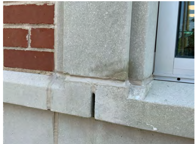
Cast Stone Jamb Repair and Sealant
