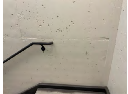
Concrete Wall Finish in Stair
