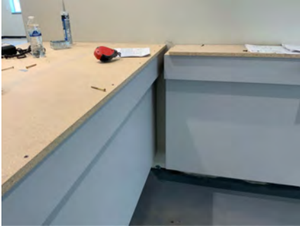
Interior Corner Gap at Reception
