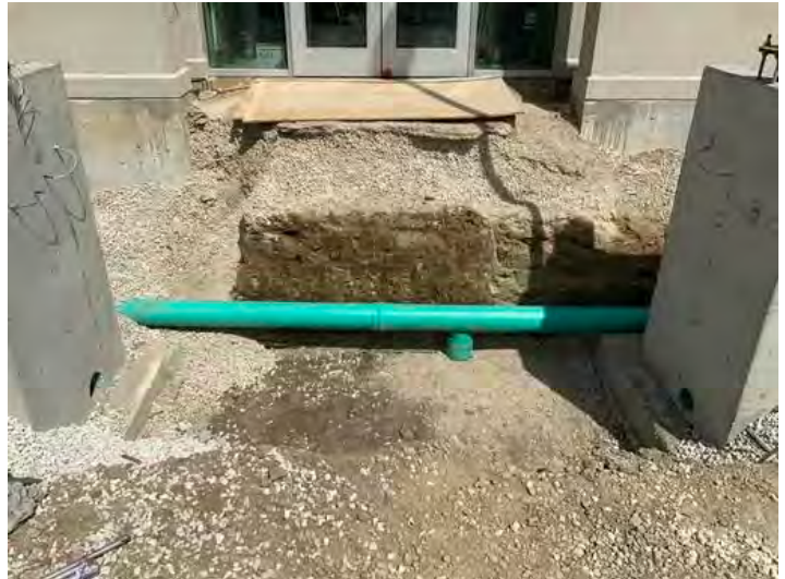
Roof drain tile being installed
