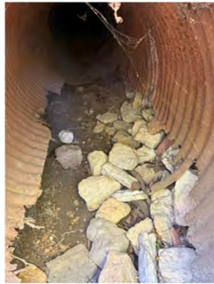
Failed Pipe Culvert
