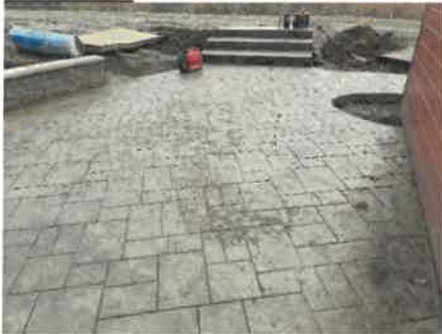
Rejected concrete slab.
