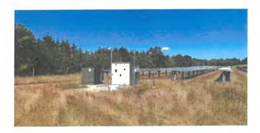
After the power is metered at the equipment pad, it interconnects into the electric utility's existing three phase distribution power distribution network. The solar installation includes a pole that houses overhead wires and leads to another pole that is controlled by the electric utility. All 5MW of community solar will have a single point of interconnection.
