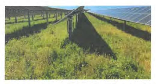
The racking system is attached to driven I-beam that secures the installation to the ground. The I-Beam is driven directly into the ground. The racking and footings are within accepted professional standards given the local soil and climate, and are professional engineered to withstand winds exceeding 150 MPH.
