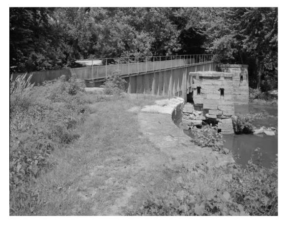
The earliest Aqueduct at Aux Sable Creek, built as part of the I & M canal project, was a timber structure completed in 1847. This structure was replaced with the present riveted steel trough in 1927.
