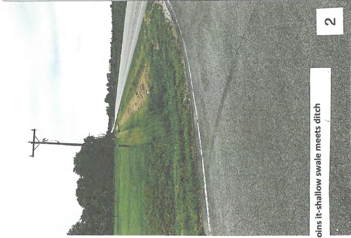
Parks Property-note gentle swale at road edge-yet yard muddy all the time and water traveling north to the Casey property
